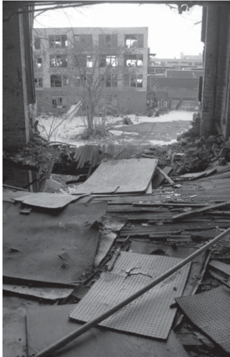
Scrapper has created an exit from the Studebaker Corporation Complex
