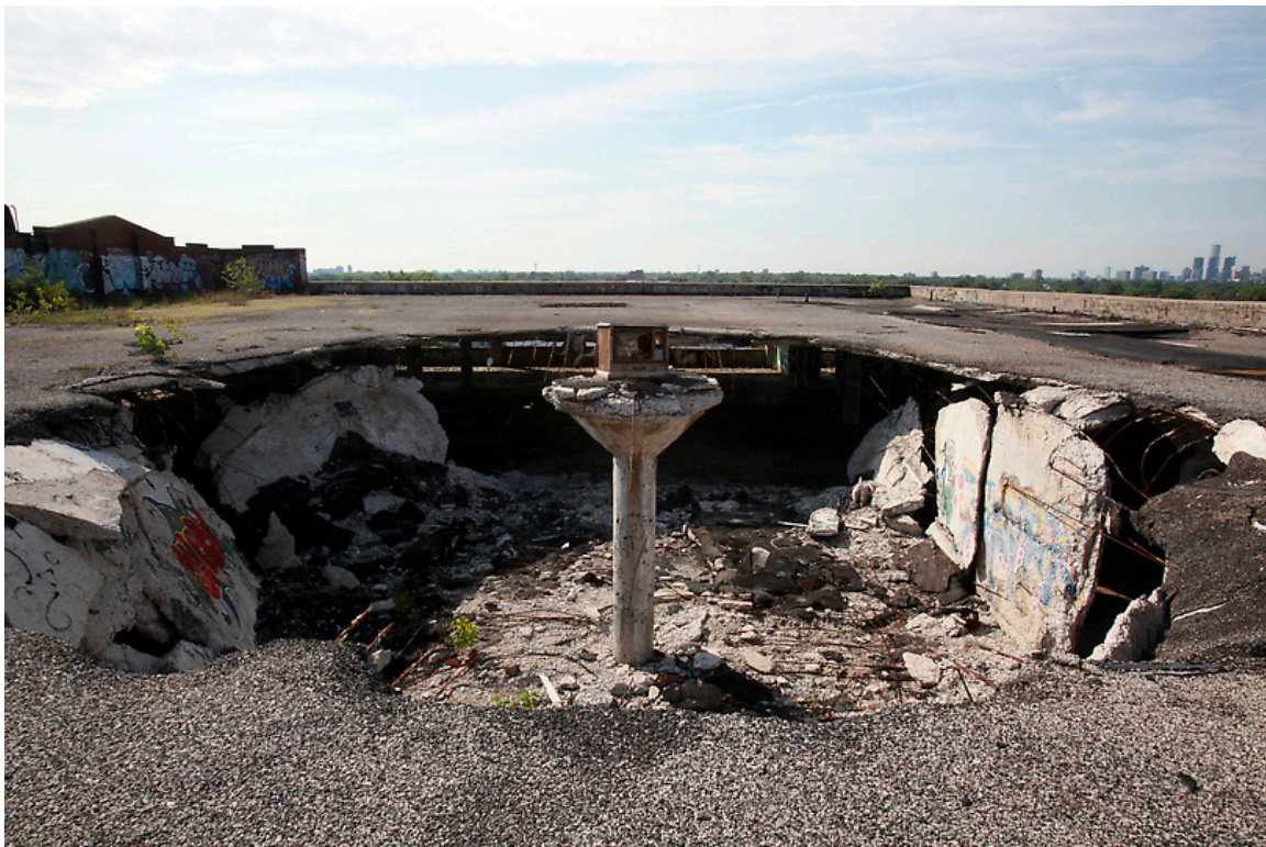
A view of the demolished Packard auto plant where Scott Hocking has the installation "Garden of the Gods," in Detroit, July 30, 2010. (Denver Post)
