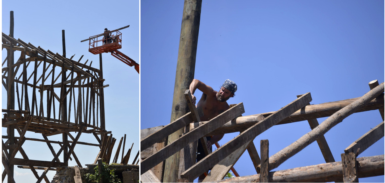
Scott Hocking puts a rafter in place from a lift high in the air. Dale G. Young
